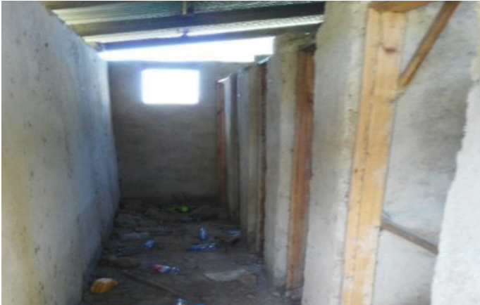
Mbeya-itiji primary school cloak room (Before)
