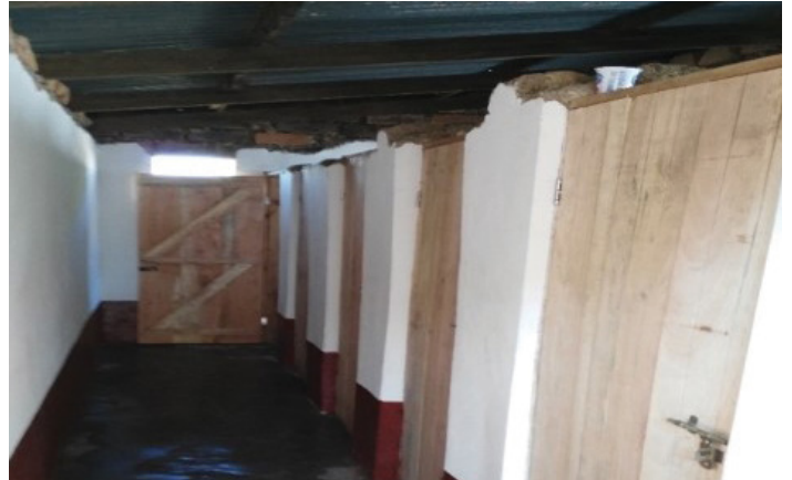
Cloak room (After)
