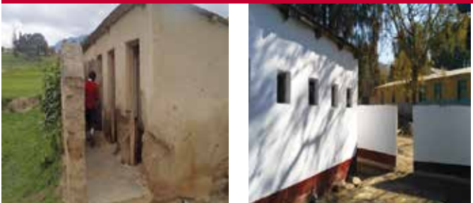
MLIMWA "B" PRIMARY SCHOOL TOILET CONSTRUCTION (BEFORE/AFTER)
