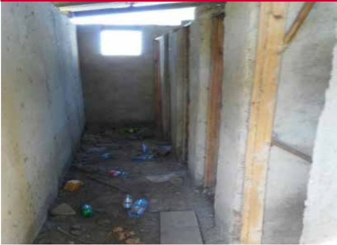
MBEYA- ITIJI PRIMARY SCHOOL CLOAK ROOM (BEFORE)
