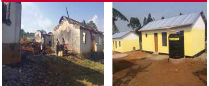
KATERERO PRIMARY SCHOOL TEACHERS HOUSES (BEFORE/AFTER)
