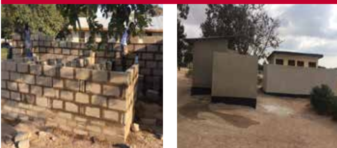
MADENGA PRIMARY SCHOOL TOILET CONSTRUCTION (BEFORE/AFTER)
